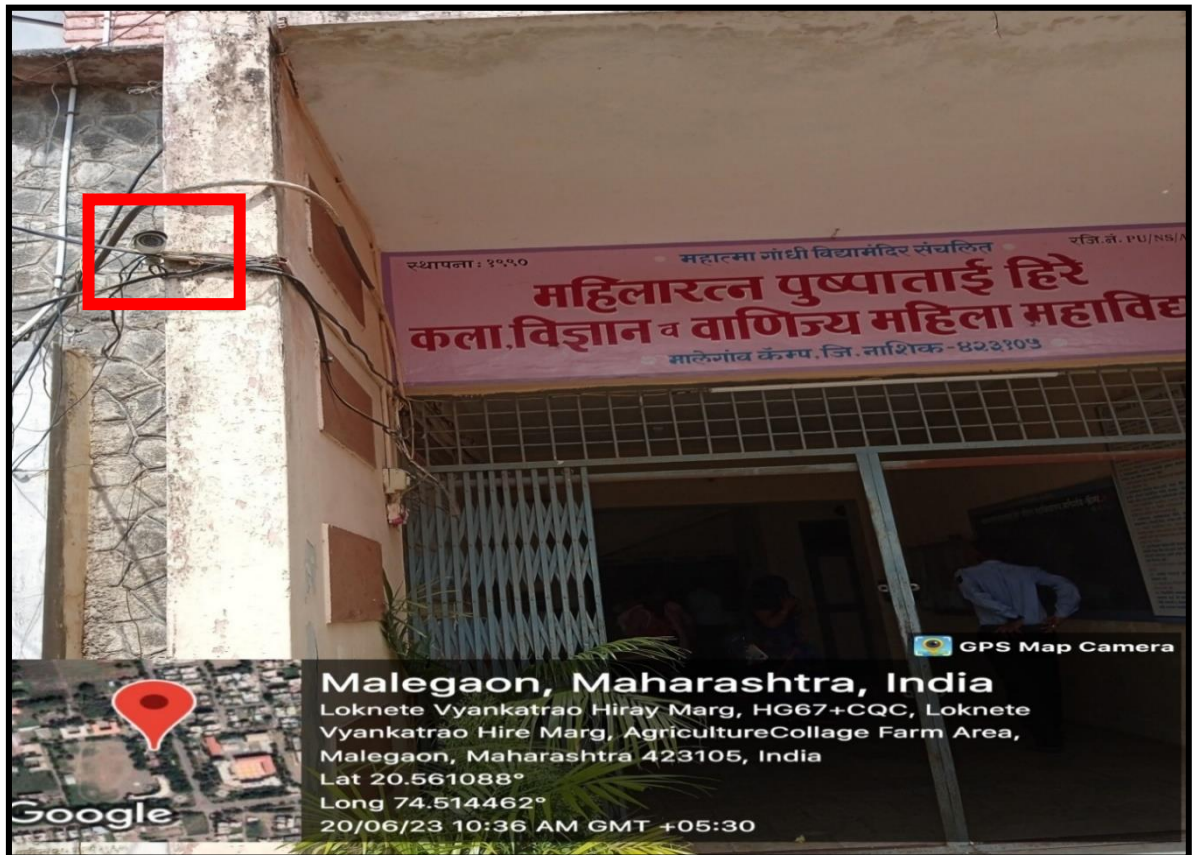
CCTV Camera in college entrance
